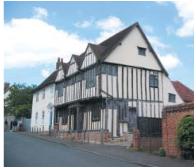
Shilling Grange. Built 15th c., refaced 18thc., derelict early 20thc., restored 1930-
