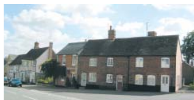
Cottages, High Street
